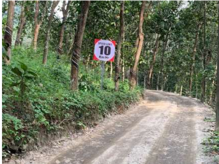
Figure 5: Photograph of Access Road to Quarry
